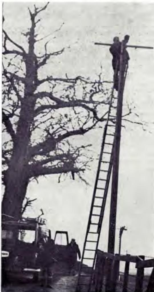
MANWEB linesmen at work on the spur line through Delamere Forest after trees crashed down on the conductors.
